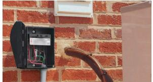
Eaton's updated ACD features a modern-looking side-hinged door for easier access to the disconnect.
